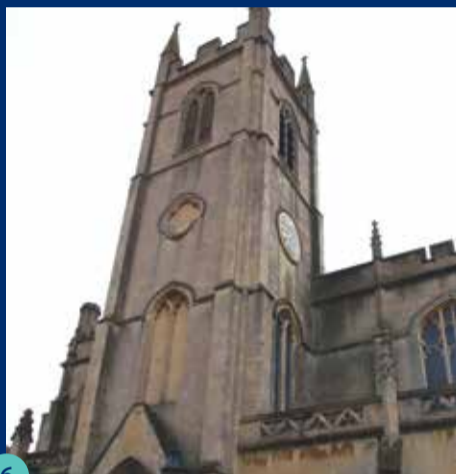
6 Christ Church Julian Road. 1798 Architect: John Palmer
