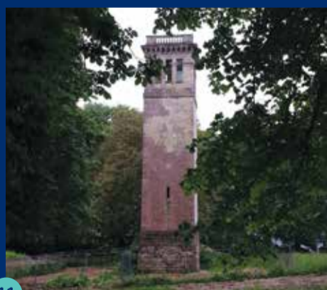
11 Blaine's Tower, Hamilton Road. c.1870*
