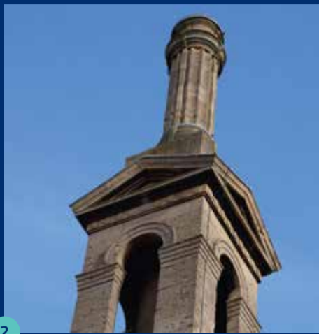
2 Bath City Laundry chimney. 1887-8 Architect: Charles Edward Davis
